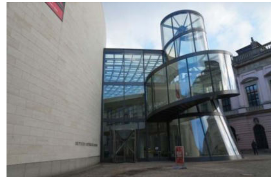
Elevator in the New Building of the German Historical Museum
